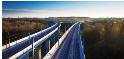
Sud Europe Atlantique High Speed Line (SEA HSL), France
