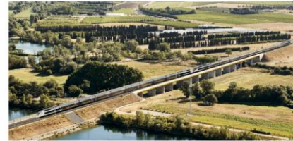
High Speed Line Nimes-Montpellier (CNM), France
