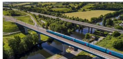
High Speed Line Bretagne-Pays de la Loire, France
